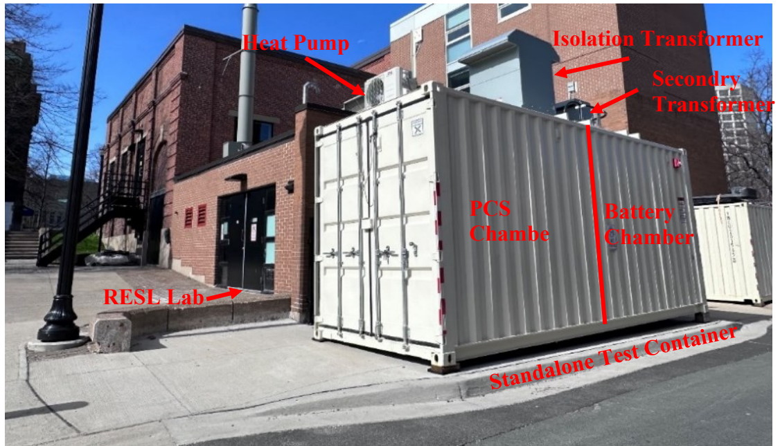
Figure 4.8: RESL Standalone Test Chamber
