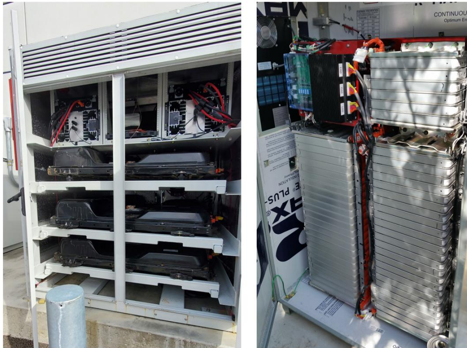
Figure 3.12 Examples of pack-level (left) and module-level (right) repurposing of Nissan Leaf EV batteries in second-life energy storage applications.
